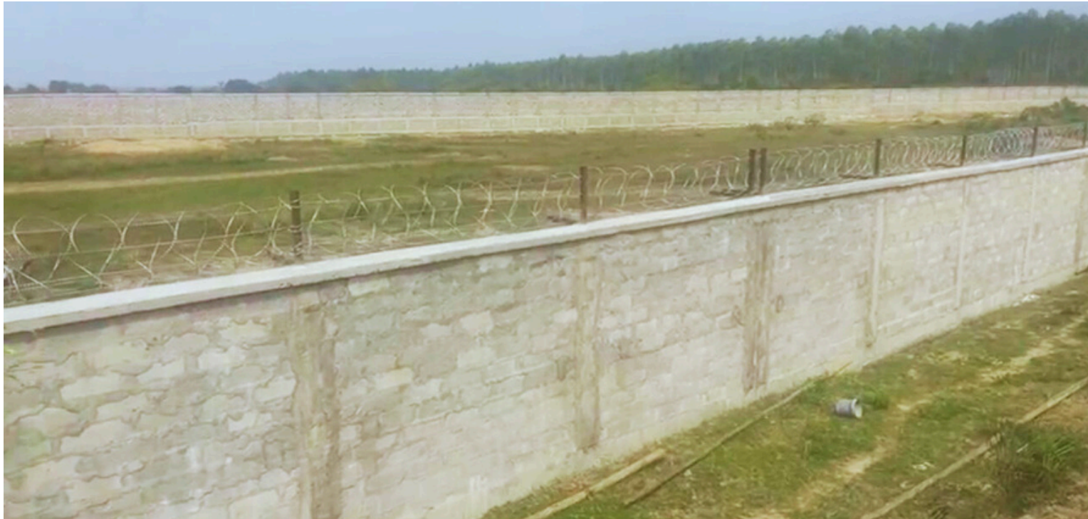
5000 Meters (12 Ft) Compound Wall at Tada - One Stop Warehouse
